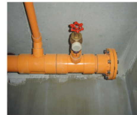
Angle valve connection and test valve piping
