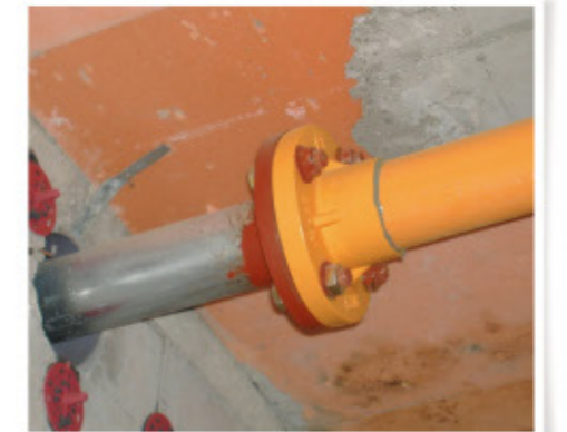
Connection with other piping (valve socket and flange connection)
