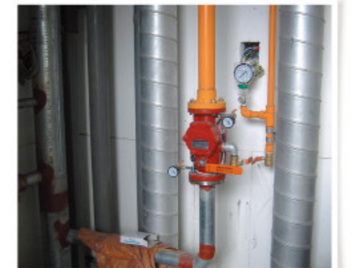
Angle valve connection and test valve piping
