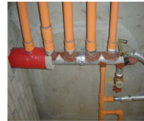
Connection with other piping (valve socket and flange connection)
