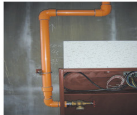
Second alarm valve and fire hydrant box
