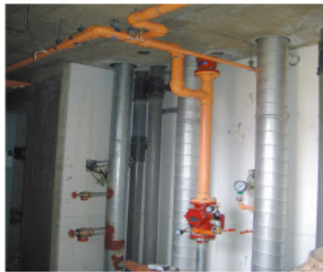
Second alarm valve and fire hydrant box
